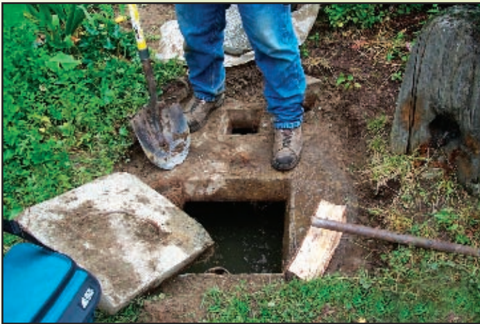
Septic tank baffle screen inspection in progress
