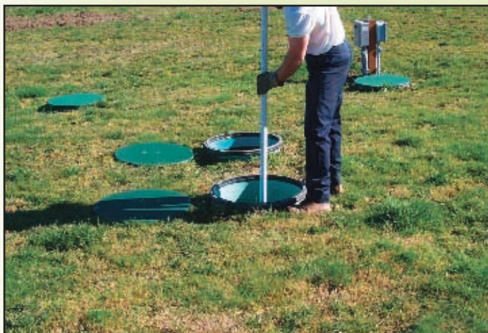
Septic tank inspection in progress
